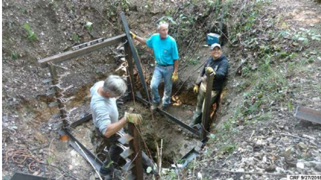
Work on a cupola gate on Radium Cave.
