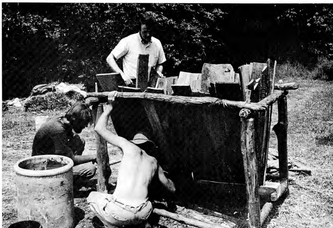
Figure 16. (a) Construction of saltpetre vat. (b) Removing niter earth from Mammoth Cave.
