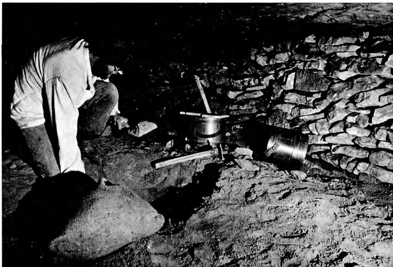
Figure 16. (a) Construction of saltpetre vat. (b) Removing niter earth from Mammoth Cave.
