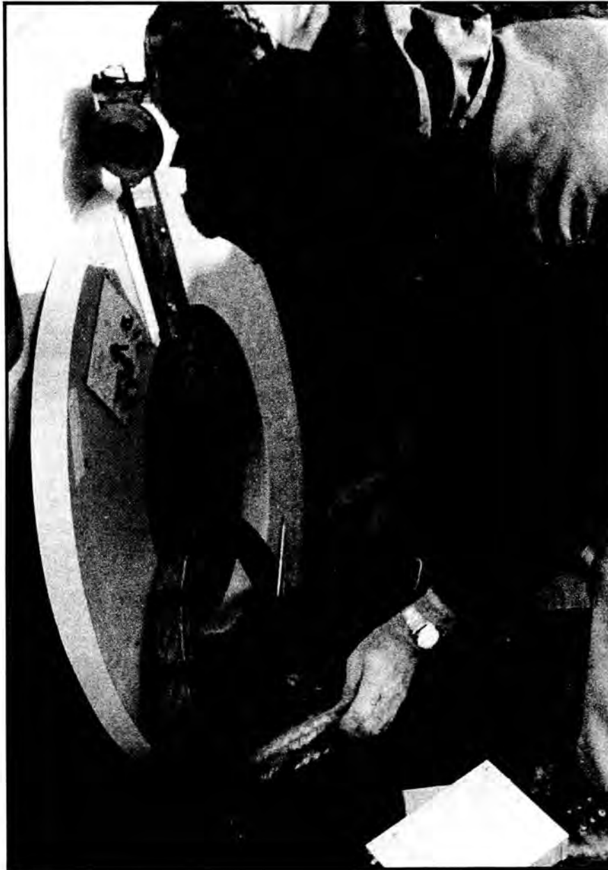
Figure 2: Father Paul Whiteman checks his cave transmitter prior to sending it into Fitton Cave to mark radio locations. Note the inclinometer on the large surface receiver loop antenna which was used to estimate the transmitter depth below the surface location. (Photo by Pete Lindsley).
