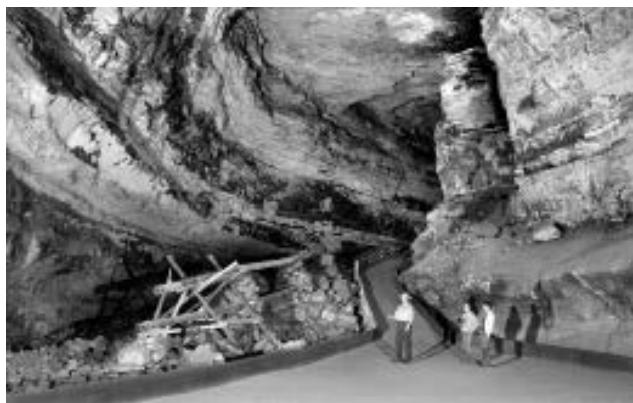
**Figure 9:** Pipes constructed from hollowed-out tulip tree trunks to convey water from the entrance and nitrate-rich liquid back to the surface (~1812).
